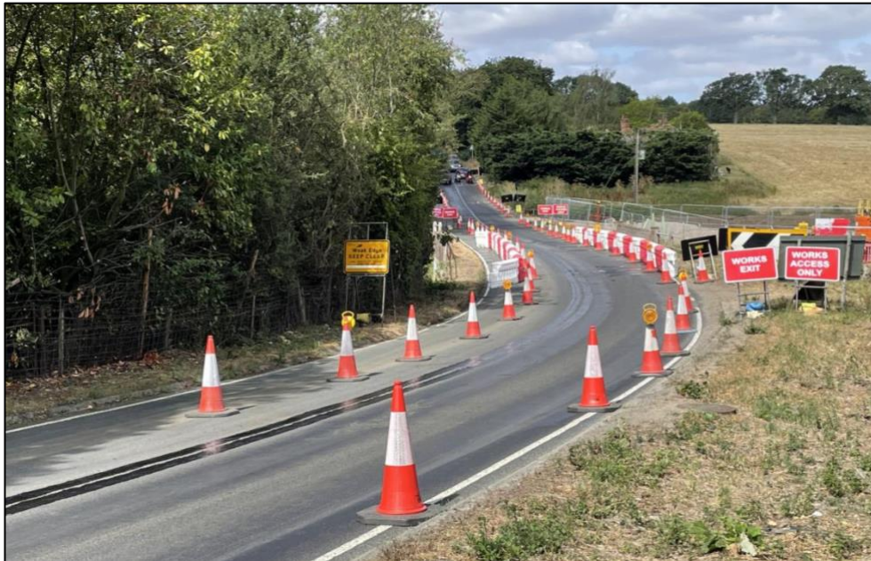
Work started on the bridge in July 2026
